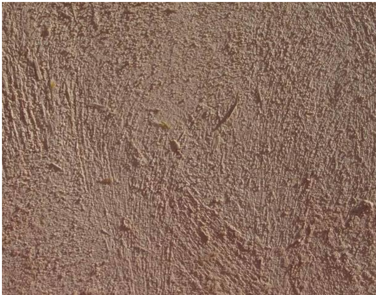
Fig. 28: Image of a plastered wall using the straw-mud mixture.
