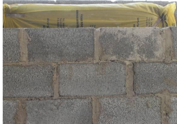
Figs. 33-34: Polystyrene is used here for insulation in wet construction (left), while rockwool is used for insulation in dry construction (right).
