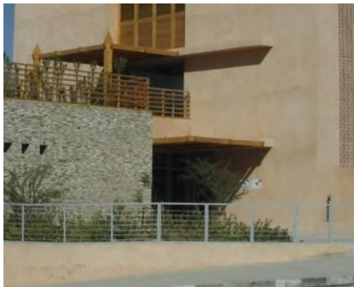
Figs. 6-9: Images of different shading elements used in the building to shade external walls and openings.
