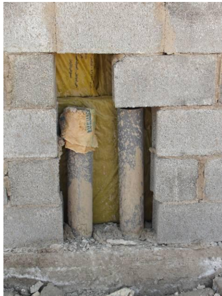
Fig. 13: Image showing the inlet for the underground pipe while under construction.
