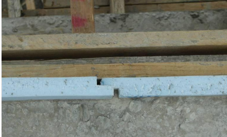
Fig. 31: Image showing the overlapping of insulation material to insure equal distribution.
