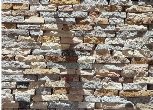
Fig. 25: Image showing the stone cladding pattern produced using leftovers from stone workshops.
