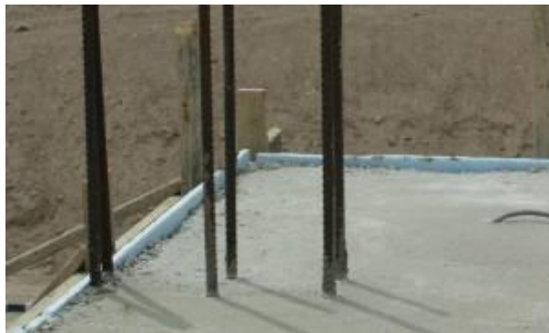
Figs. 29-30: External edges of floor slabs insulated by polystyrene strips are used to avoid the formation of thermal bridges.
