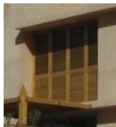
Figs. 6-9: Images of different shading elements used in the building to shade external walls and openings.
