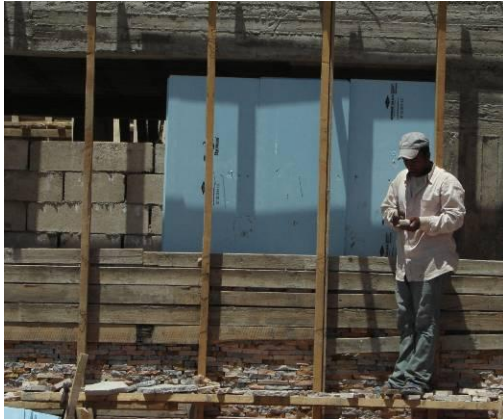
Figs. 33-34: Polystyrene is used here for insulation in wet construction (left), while rockwool is used for insulation in dry construction (right).
