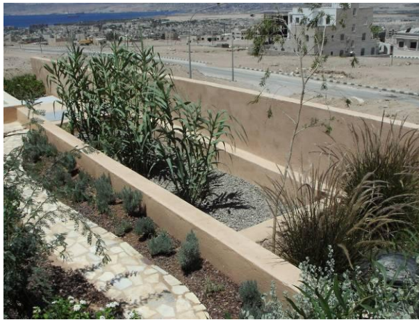
Fig. 51: Artificial wet land with bamboo (left) and settling barrel (bottom right).
