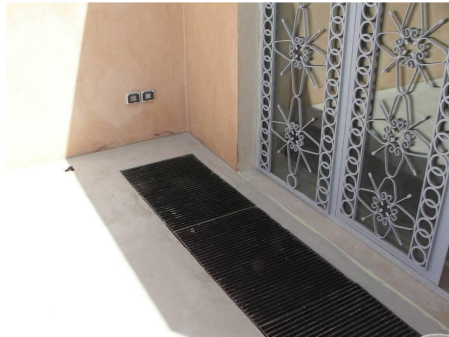
Figs. 10-11: Section and image showing the evaporative pool and its cooling effect on the air that enters the kitchen door.
