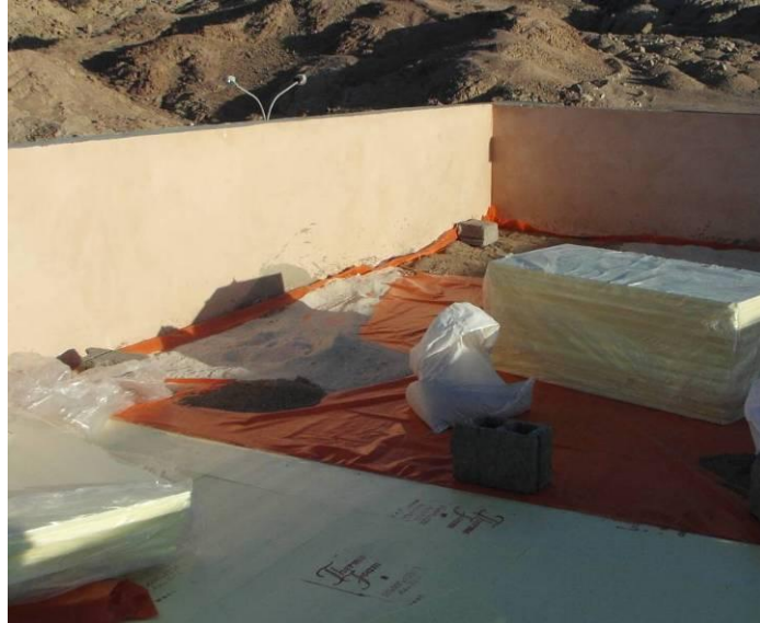
Fig. 36: Image of polyethylene sheets spread over the roof.
