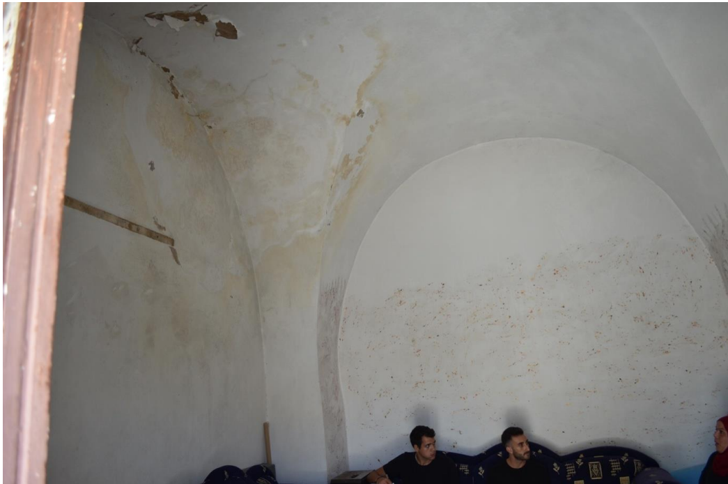
House 2, view of the remaining vaulted room.
