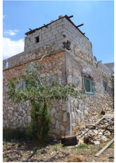
House 3, back view.
