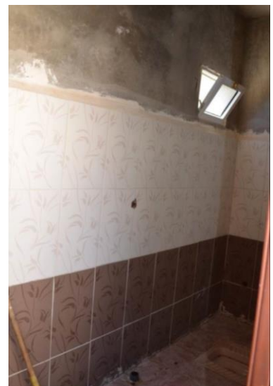
House 4, view of the bathroom.
