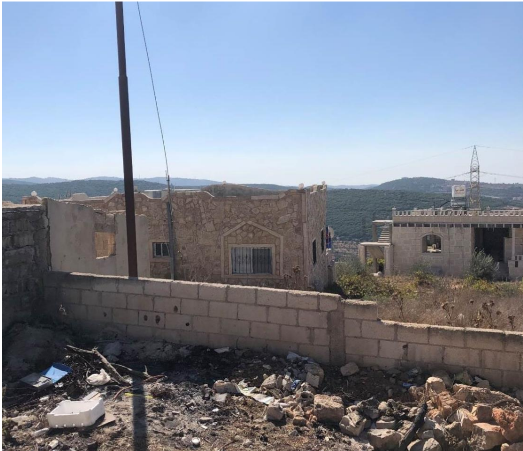
House 6, back view.
