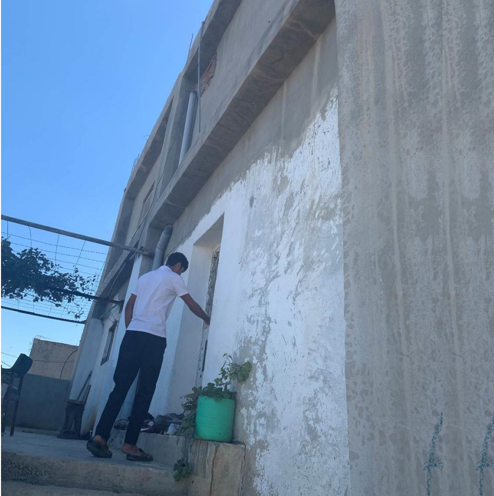
House 13, entrance view.
