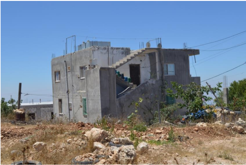
House 5, view of the northern and eastern elevations.
