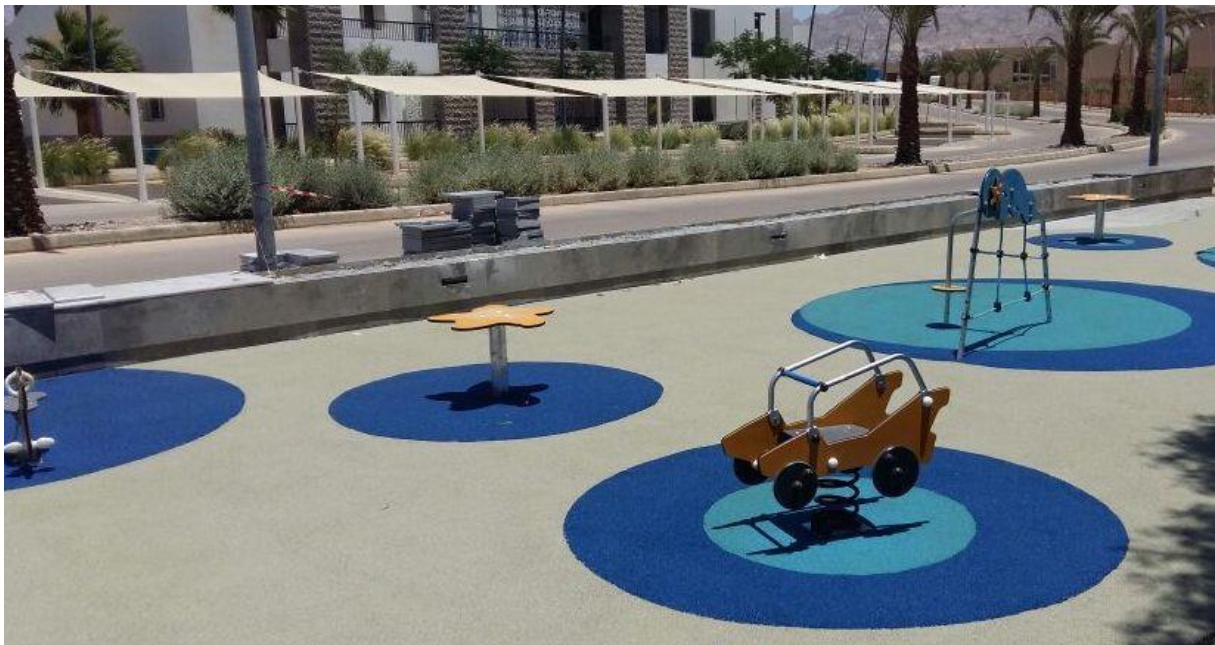
Poured rubber surfacing in a playground in a resort in Aqaba. Photo by Lara Zureikat.
